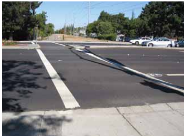
CROW CANYON ROAD CROSSING
