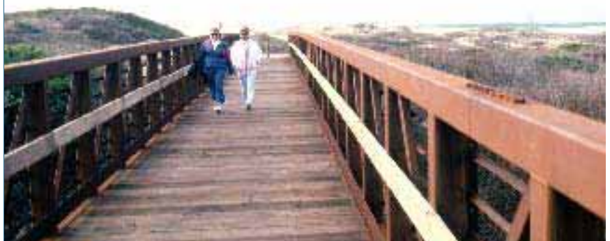
JOHN HERNANDEZ BRIDGE
