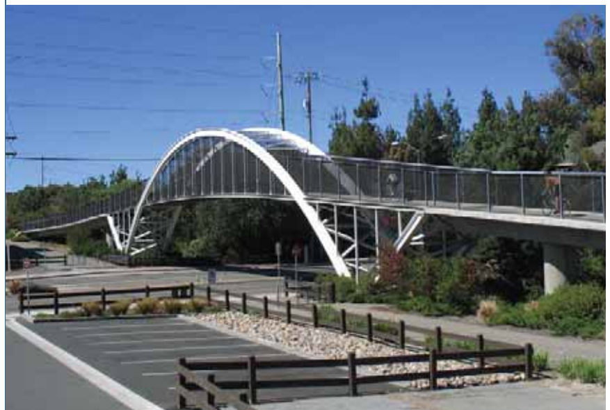
OVERCROSSING AT YGNACIO VALLEY ROAD
