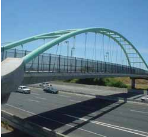
BERKELEY I-80 PEDESTRIAN OVERCROSSING
